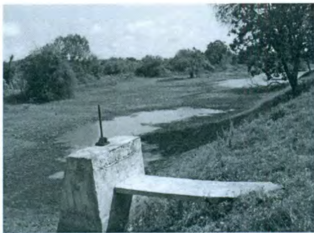
Annex Figure 4.1: Well Maintained Bunds of Some Rehabilitated Small Tanks in Anuradhapura District
